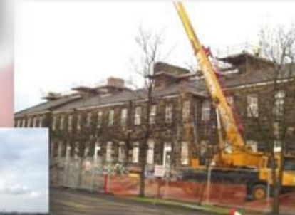
FULWOOD, PRESTON Listed Building Chimney Repairs Contract Value : £140,000
