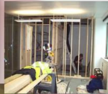
LANCASTER Office Remodelling Contract Value : £24,000
